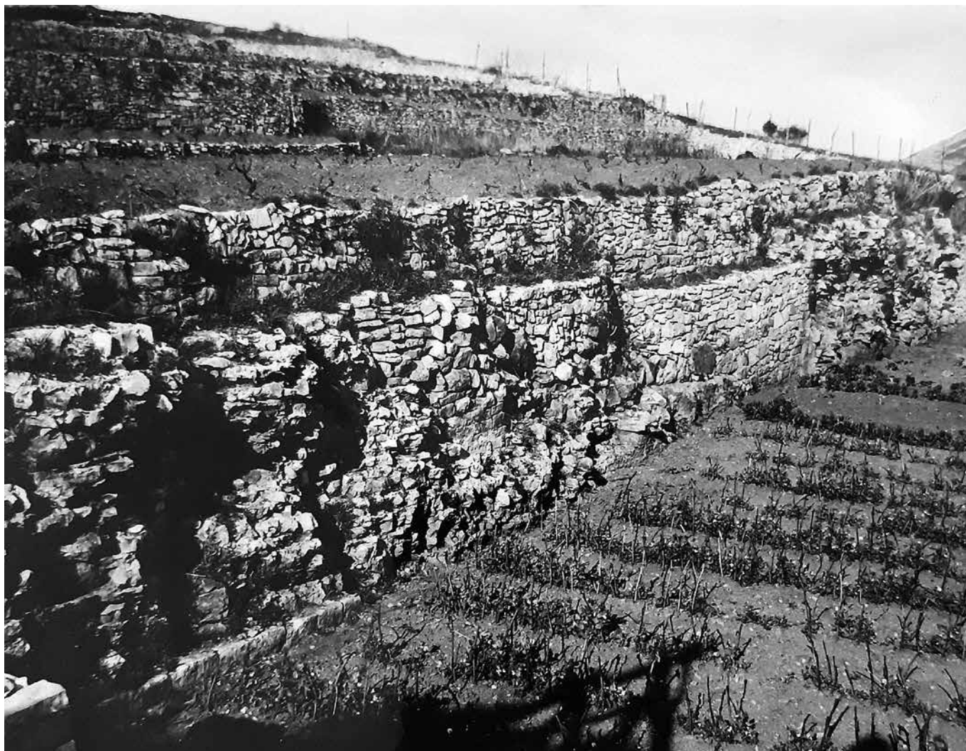
Figure 4. Supporting Roman wall with recesses, visible is the well-preserved base of the wall without any traces of structures to the south (Source: Archive Dyggve, negative D-1284)
